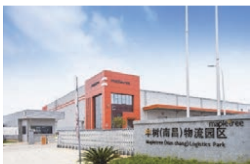
Mapletree Nanchang Logistics Park (南昌、中国) 倉庫
