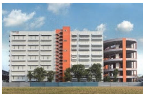
Mapletree Pioneer Logistics Hub (シンガポール) 倉庫
